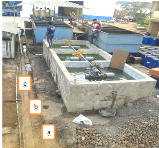
Fig. 7: Raceway ponds with single axis rotating motor constructed for fish waste water treatment., 7a. Primary treatment, 7b. Microalgae treatment and 7c. Final treated water.
